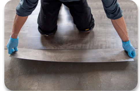
Immediate foot traffic after PSA method installation
