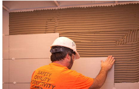
Non-slip for large tile and stone weighing up to 6 pounds per square foot used in wall applications
