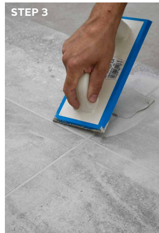
STEP 3 Proceed to grouting a minimum of 3 hours after the start of the adhesive application.
