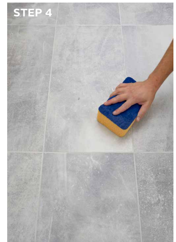
STEP 4 Clean the grout following the instructions on the grout container.
