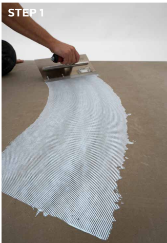
STEP 1 Apply adhesive AD-610 to an area that can be covered within 30 minutes. Give a 5 to 10 minutes flash time.
